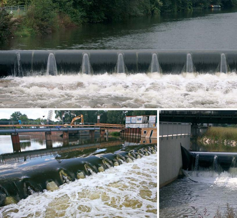
The number of **Arcon AquaPro** Rubber Dam installations is growing all the time as more engineers move away from conventional steel gate dams to flexible, safer and more reliable rubber dam systems. This trend can be seen from the rapidly increasing number of installations worldwide.
